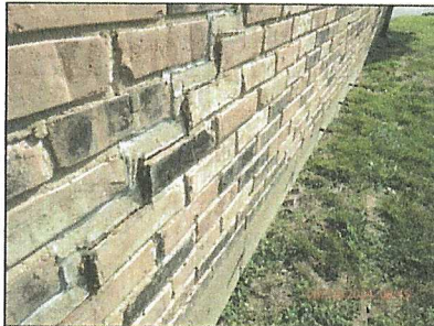
South end of building
