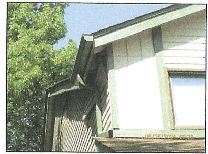
South end of building.
