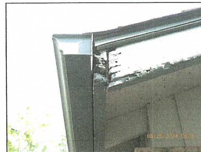
2044 - Gutter and rake boards.
