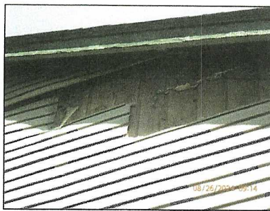
South end of building
