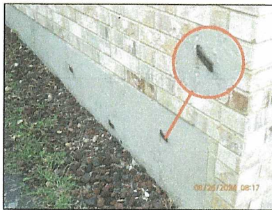
2034 - remove concrete form ties.
