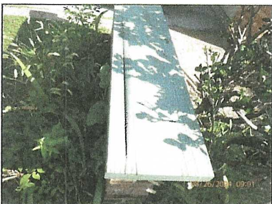
2048 - wood cap at entry wall.
