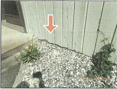
2037 Siding deterioration.
