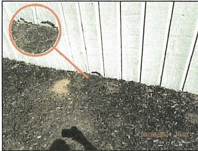
2025 - Siding deterioration.
