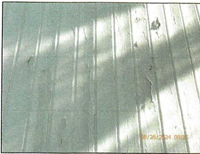
South end of building.
