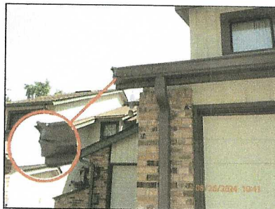
2036 - Bent/damaged gutter.
