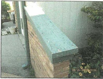
2036 - Deteriorated paint.
