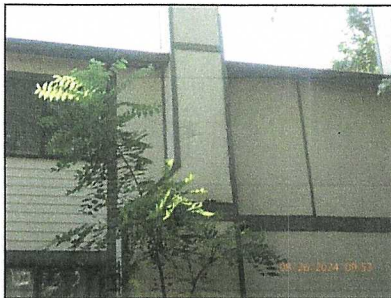
Siding at chimney.
