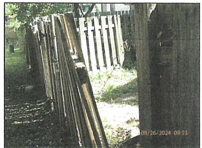
rear of building - fencing.
