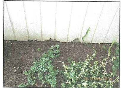
2025 - Deteriorated siding
